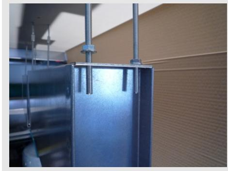
**Attach box joining sheets (Figs. 2.1 - 2.3)
